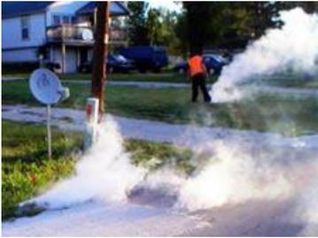
*It is not unusual to see plumes of smoke issuing up from peculiar places, such as cracks in the street, or in residential yards during smoke testing.*
