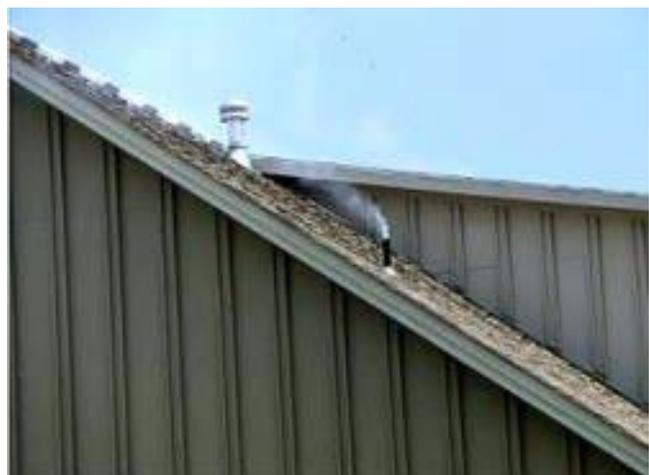
However, smoke doesn't always originate at the spot the smoke plume emerges. Sometimes smoke will escape through a defect in the sanitary sewer line, then travel or migrate along the pipe until it finds a way to rise to the surface.
